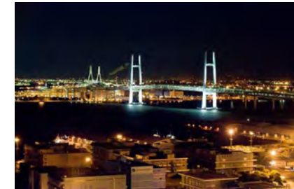
6: Yokohama Bay Bridge
